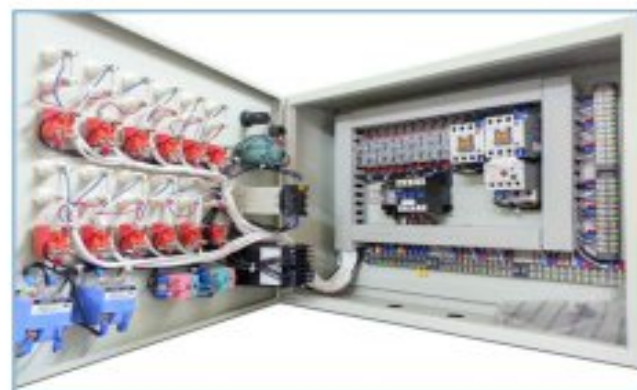
Control cabinet installation
