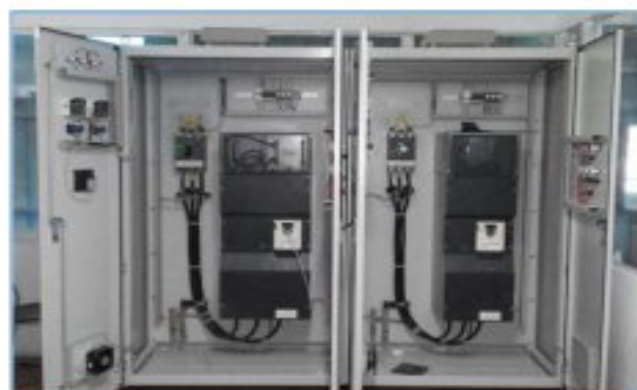
Inverter installation
